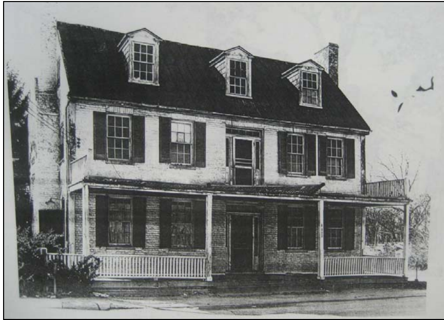
Figure 56: The George Washington House Prior to Restoration, 1972 Source: Susanna Cristofane Collection/PGCHS
