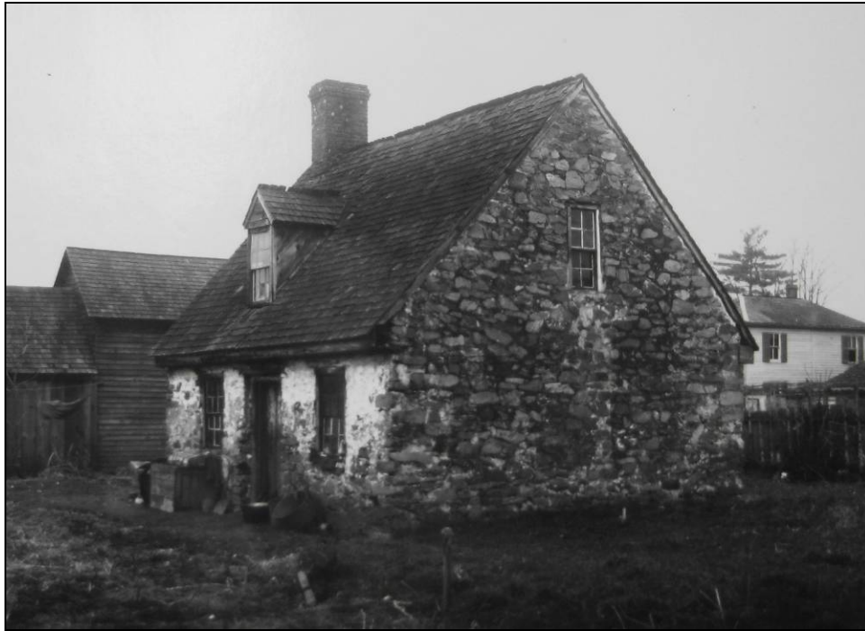
Figure 63: View of the North and West elevations of the Market Master's House, circa 1913 Source: The Rambler Photograph Collection, The Historical Society of Washington, D.C.
