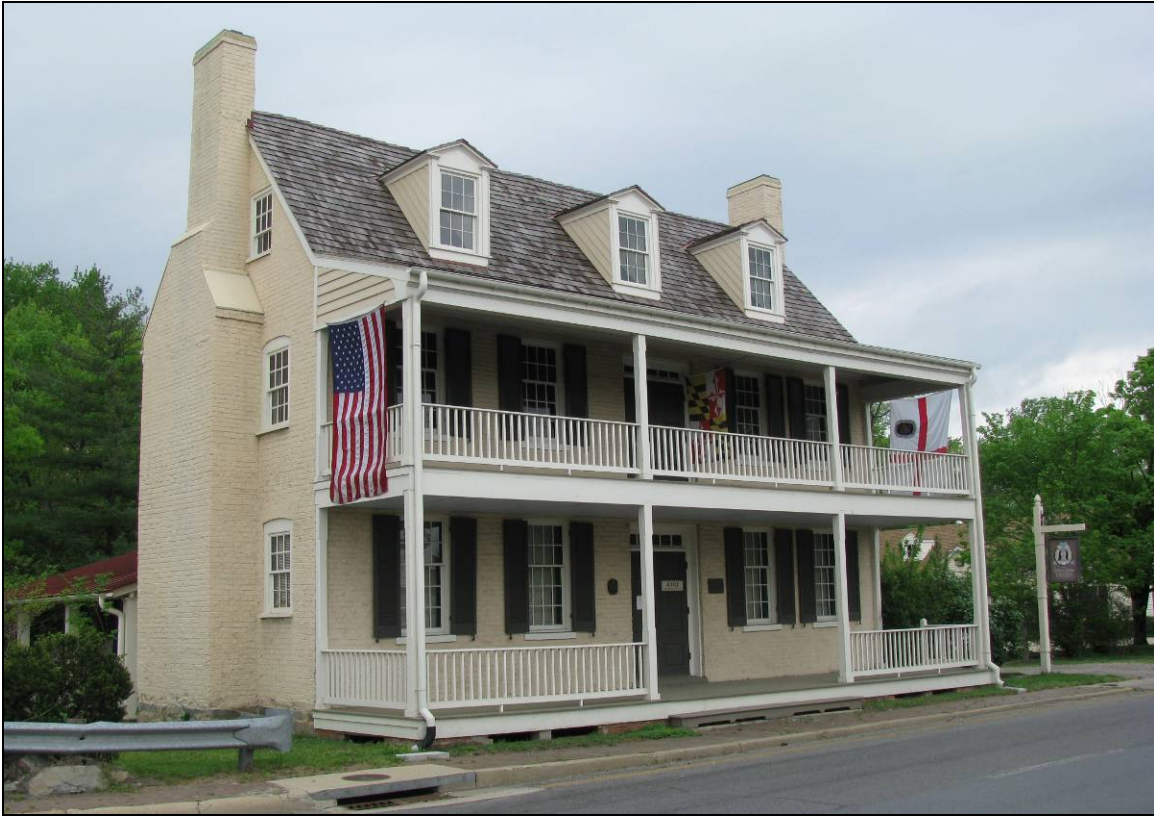
Figure 36: George Washington House View from the Southeast, 2009 Source: EHT Traceries
