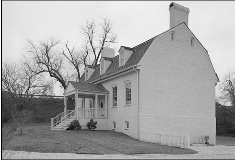
Figure 34: View of the Magruder House from the Northwest, 1980 Source: Historic American Building Survey/Library of Congress
