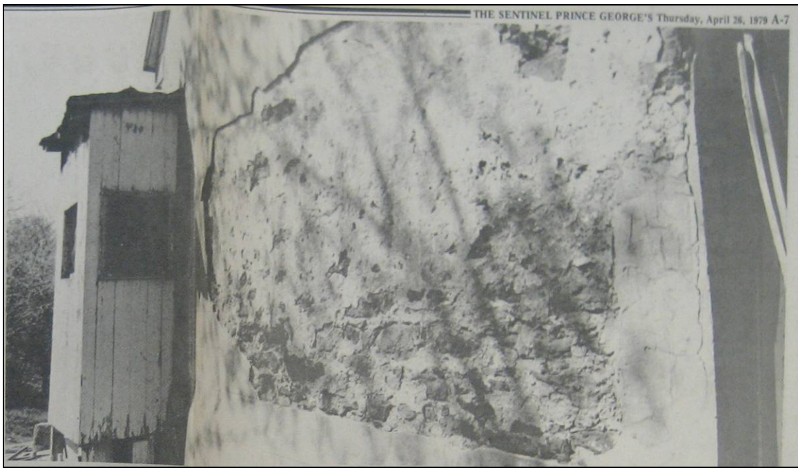
Figure 25: Exposed Stone on the Exterior of the Magruder House, 1979 Source: The Prince George's Sentinel/PGCHS Library
