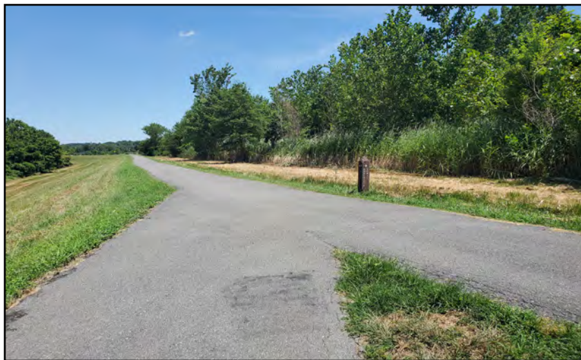
Anacostia River Trail - Asphalt Surface
